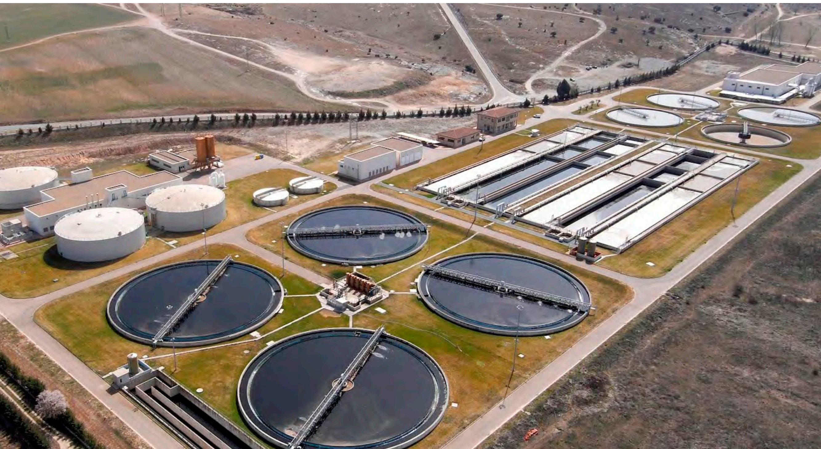
Salamanca Wastewater Treatment Plant.
